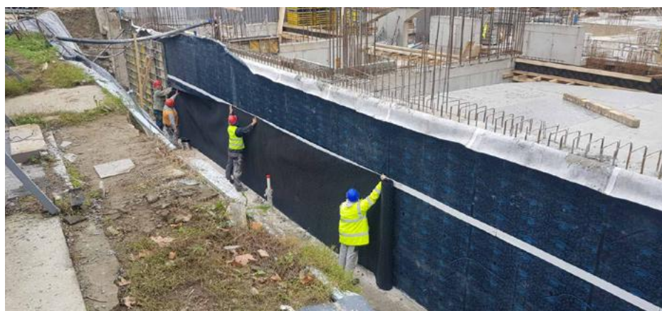
► Posa membrana AMPHIBIA in verticale
