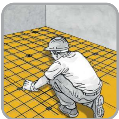
Placing reinforcement mesh
