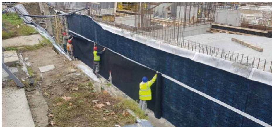
➤ Vertical application on formworks
