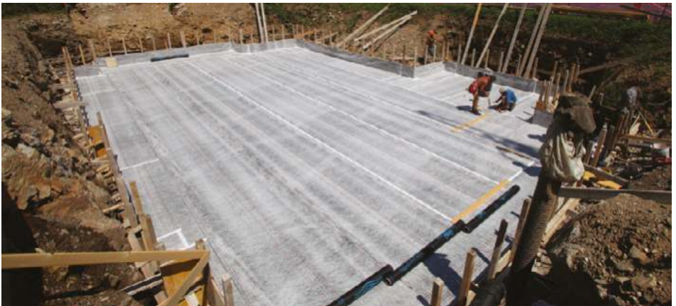
► Raft foundation with AMPHIBIA system
