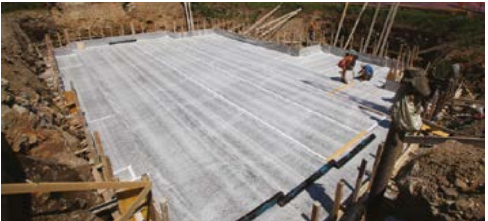
► Raft foundation with AMPHIBIA system
