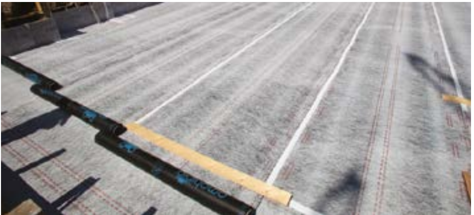
► Raft foundation with AMPHIBIA system
