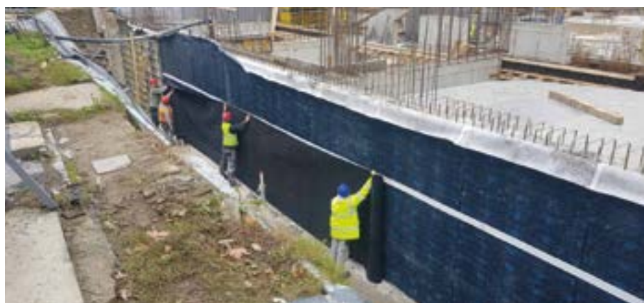
➤ Vertical application on formworks
