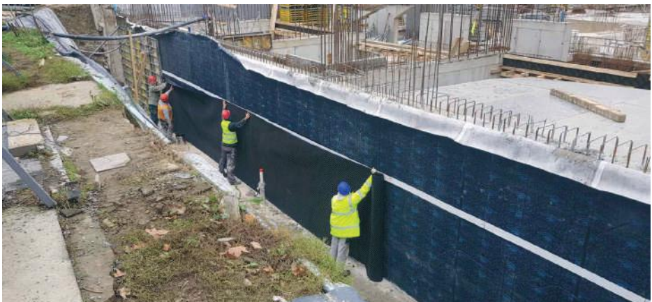
> Vertical application on formworks
