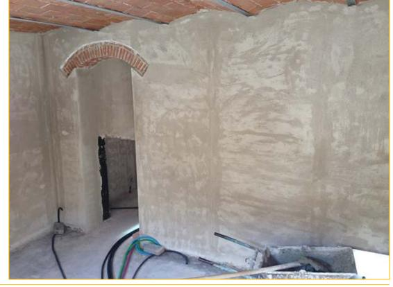
CALIBRO NHL is a Natural Hydraulic Lime NHL plaster, according to EN 459, eco-compatible, suitable for damp-proofing, salt-resistance and anti-condensation treatments on any type of damp wall, both
