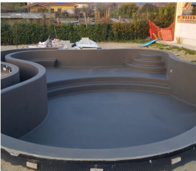
Example of waterproofing inside the structure
