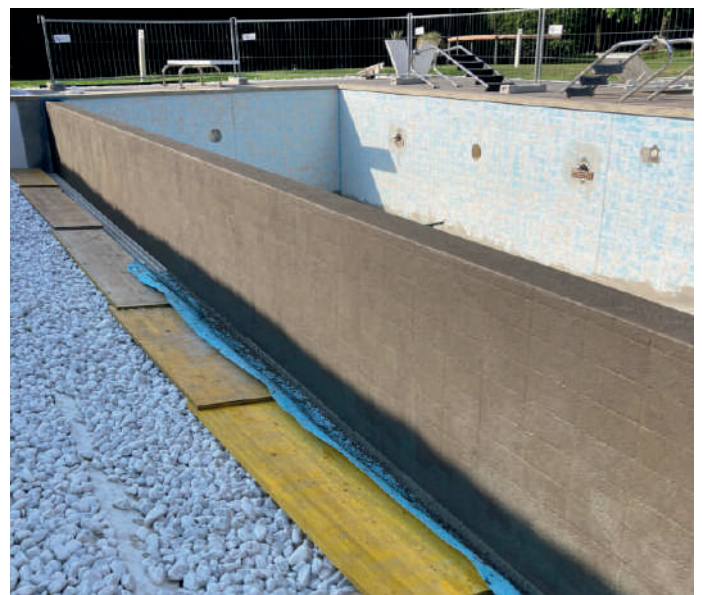
Example of waterproofing outside the structure
