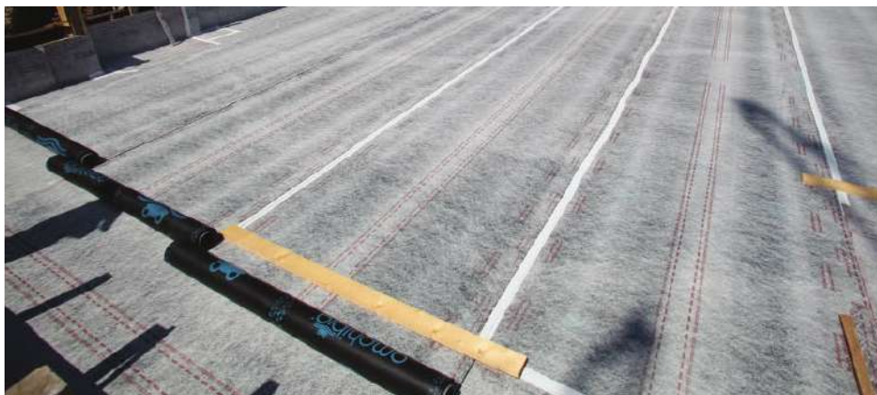
› Raft foundation with AMPHIBIA SYSTEM
