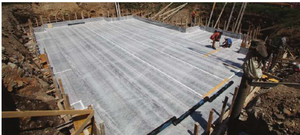
› Raft foundation with AMPHIBIA SYSTEM
