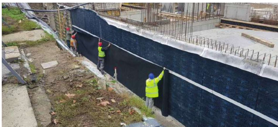
› Vertical application on formworks
